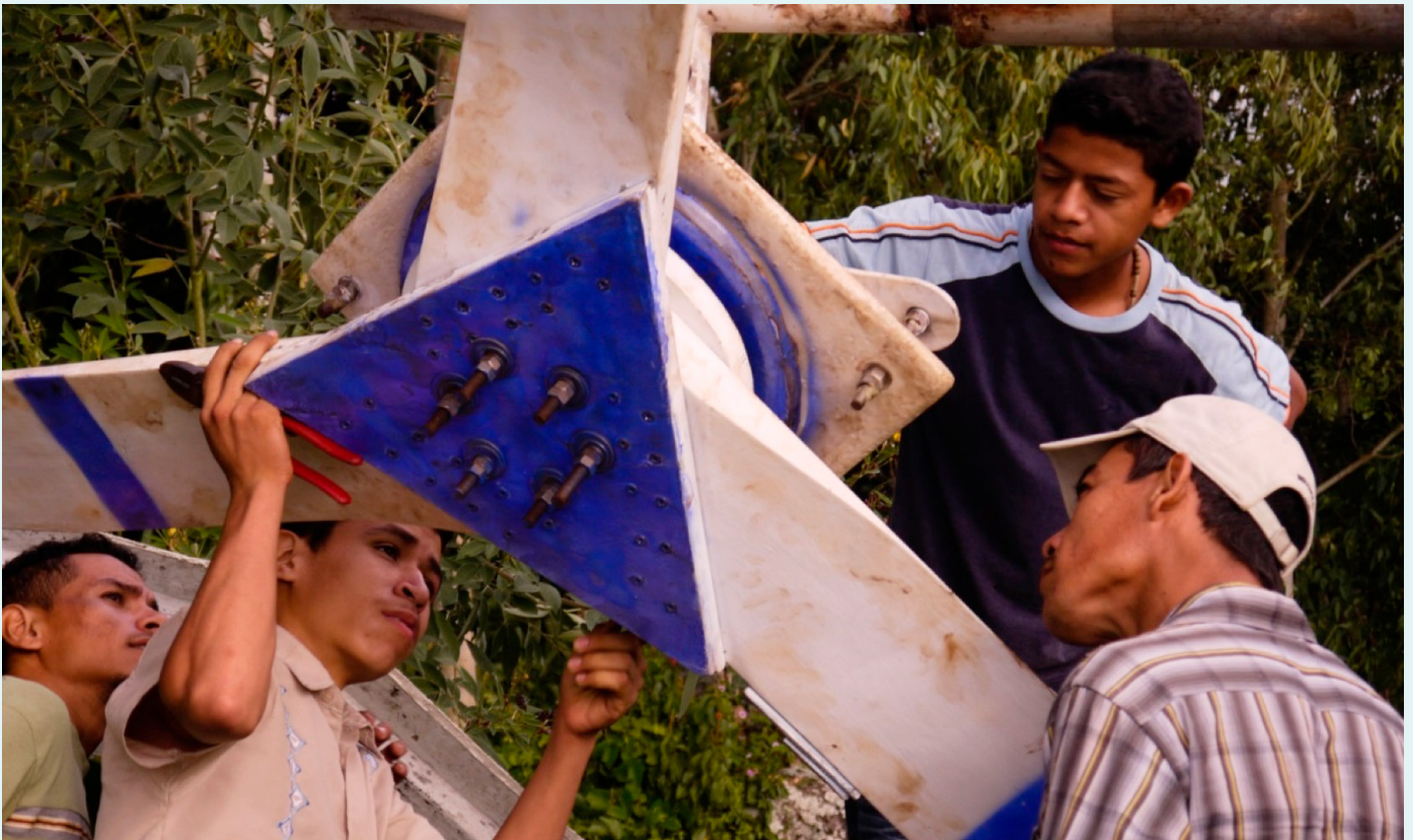
Figure 4 – Inspection of the rotor and stator to prevent a potential future failure by the motivated and capable Cuajinicuil technicians. Photo by Jon Leary
