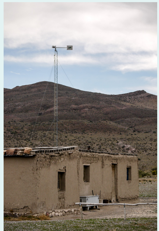
Figure 6 – a) A commercial maintenance team in the Falklands carries out a routine annual service on one of the islands' many SWTs (left); and b) a SWT stands still in remote rural Patagonia after the blades fell off and the state-run centralised maintenance team were unable to send anybody to fix it (right). Photos by Jon Leary.
