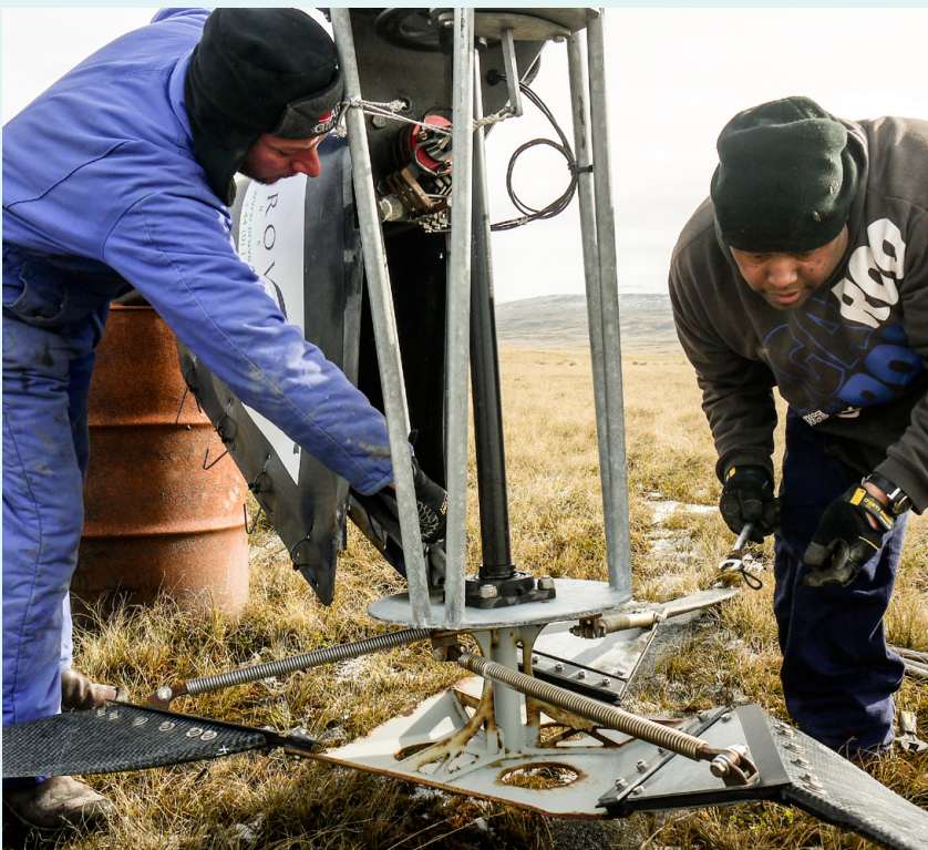
Figure 6 – a) A commercial maintenance team in the Falklands carries out a routine annual service on one of the islands' many SWTs (left); and b) a SWT stands still in remote rural Patagonia after the blades fell off and the state-run centralised maintenance team were unable to send anybody to fix it (right). Photos by Jon Leary.
