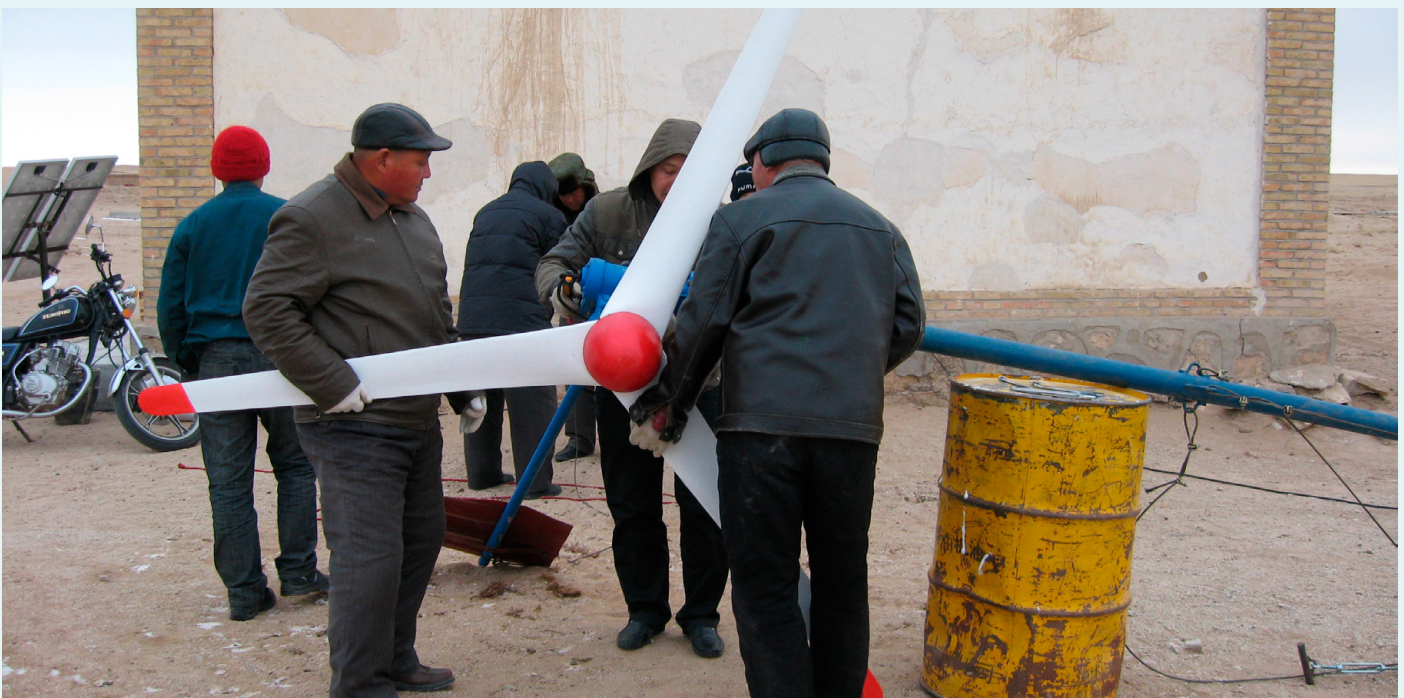
Figure 3 – A group of end-users installing a SWT in IMAR, China in 2009 (photo by Long Seng To).
